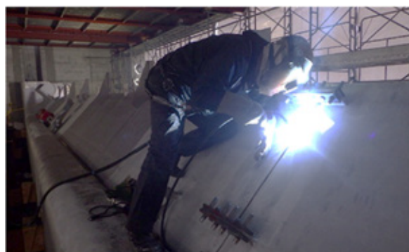
写真-15 扉体溶接
